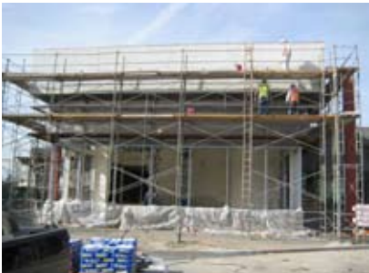
Workers install drywall, glazing and stucco on the new facility.
